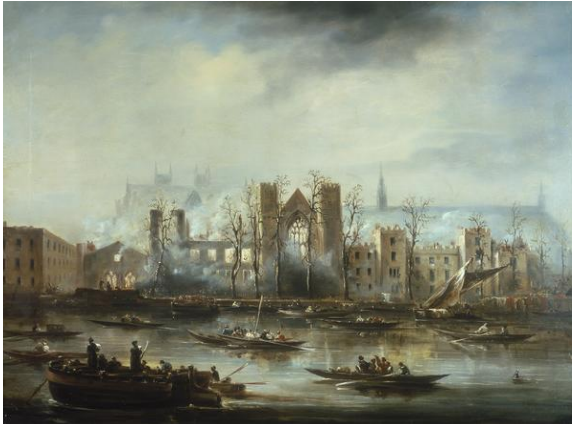
End of the Fire
